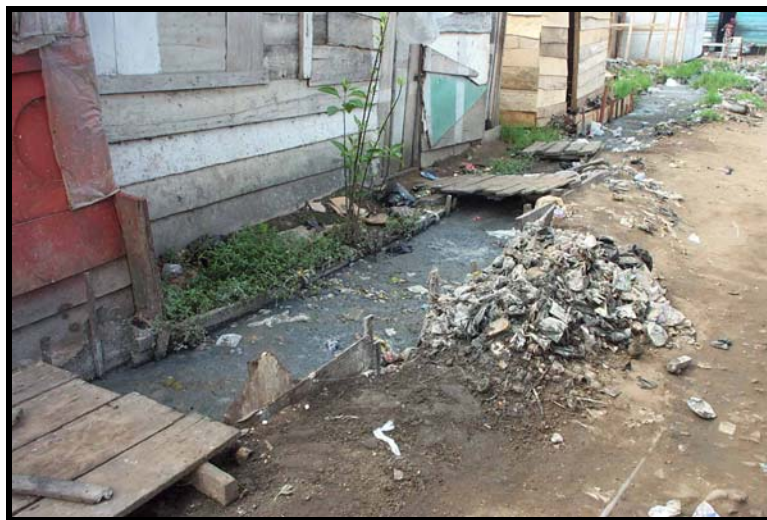
Figure 30: Conditions of storm water drains several weeks after rains
