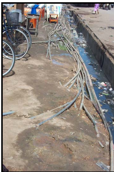
Figure 7: Bundled small diameter water main supply on Abosseyokai Road
