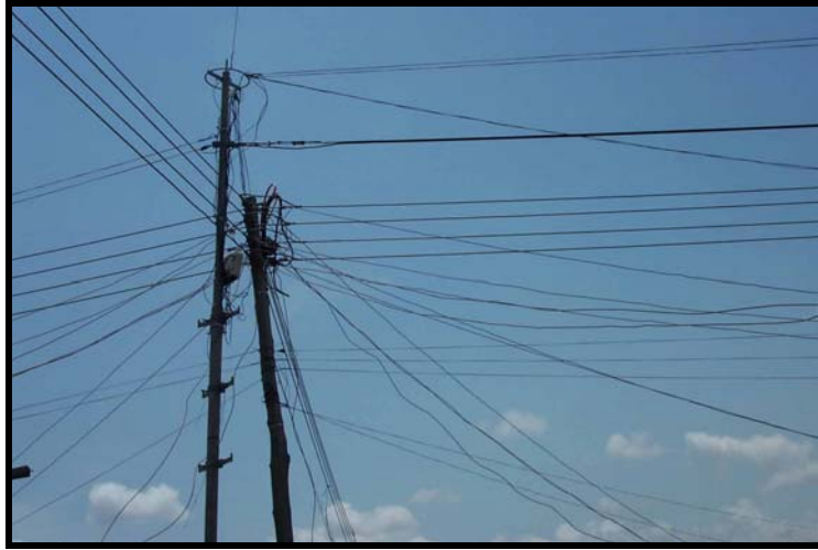
Figure 18: Random electricity distribution with both legal and illegal connections
