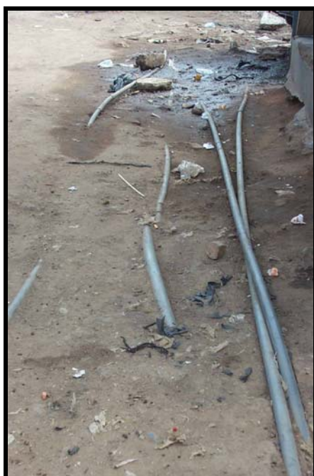
Figure 6: Water mains laid on the surface
